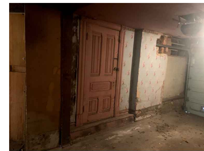
FIG. 1: EXISTING DOOR IN GARAGE COVERED BY SIDING
